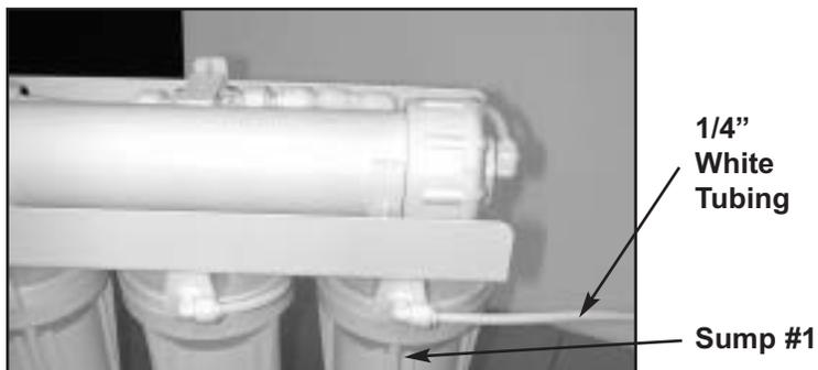
a. Connect the 1/4" white tube to the elbow of sump #1. The other end of the elbow should be connected to inlet saddle valve. Refer to inlet saddle valve installation on page 6.
