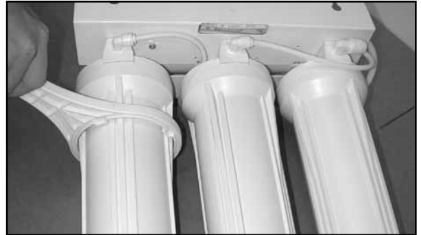
Figure 11 - Using sump wrench to change filter cartridges
