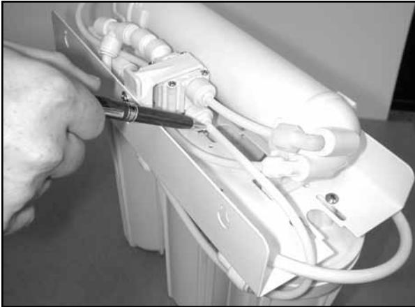
Figure 9 - Disconnect pre-carbon outlet tube from shutoff valve
