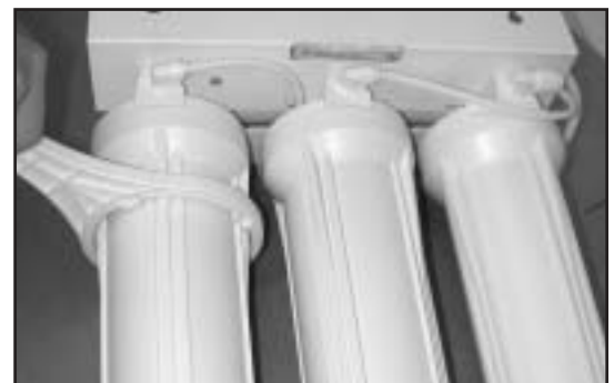
Figure 11 - Using sump wrench to change filter cartridges
