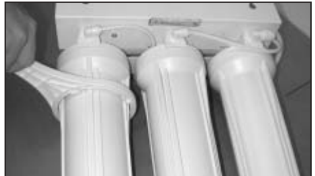
Figure 11 - Using sump wrench to change filter cartridges
